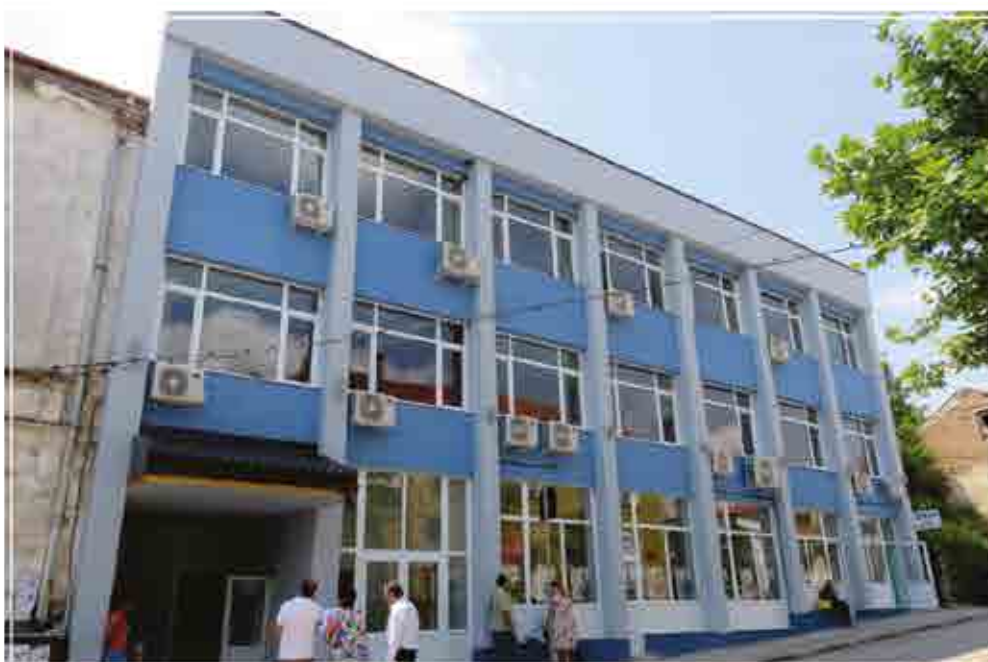
Project No 295-1 “Implementation of a package of measures for energy efficiency improvement of the Administrative building in Oryahovo”.
