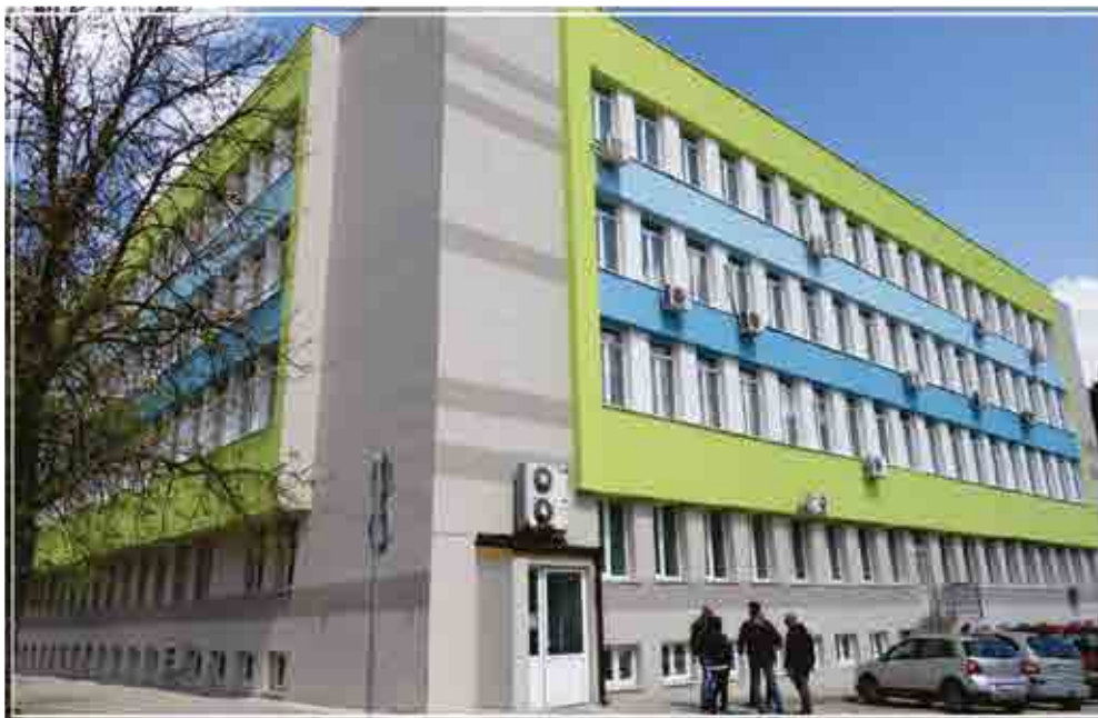
Project No 364 “Repair, modernization and implementation of energy saving measures in the building of FCF I Gabrovo EOOD - first building”.
