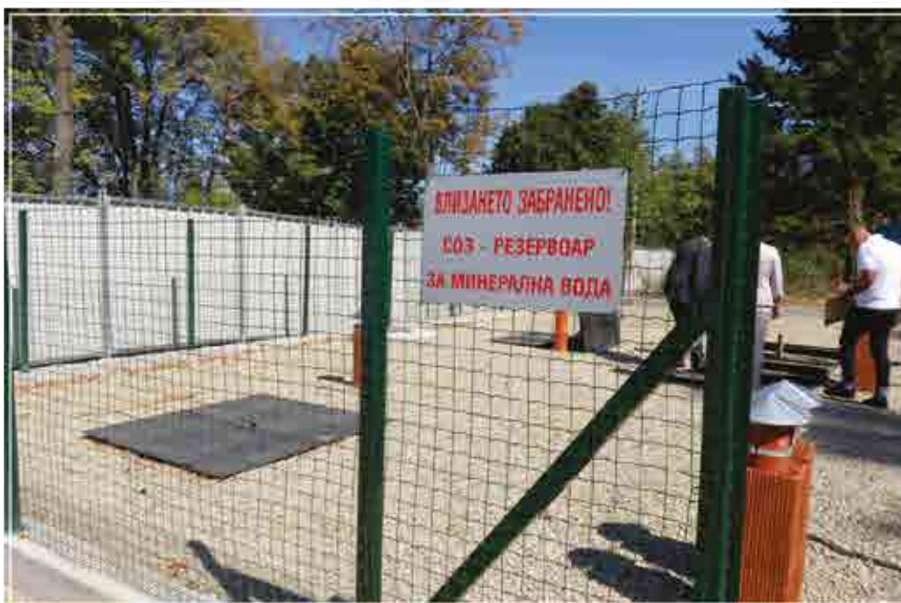
MW 003 – „Improvement and expansion of the efficient use of mineral waters from the Sapareva Banya deposit, site: Construction of a mineral water tank and supply and discharge water pipeline“.
