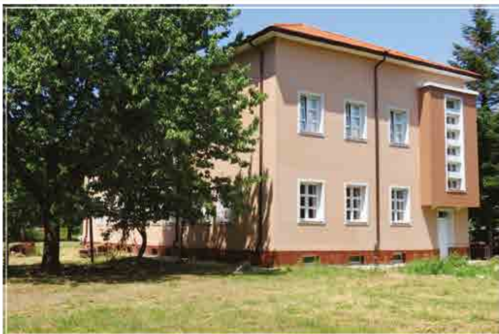
Project No 295-2 "Implementation of a package of measures for energy efficiency improvement of a health care facility in the village of Selanovtsi".
