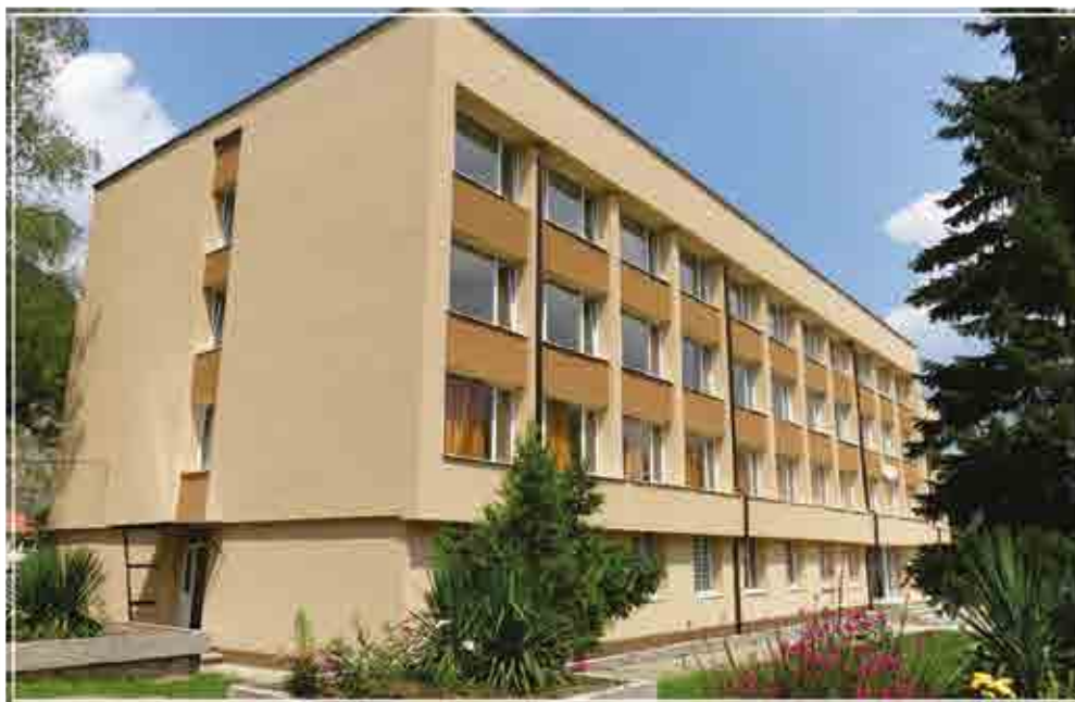
Project No 184 - Introduction of energy saving measures in Dormitory to vocational secondary school (VSS), Etropole city.
