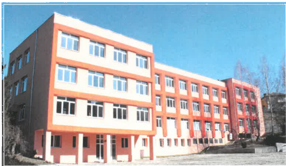
The renovated building of "Hristo Smirnenski" high school in Ardino.
