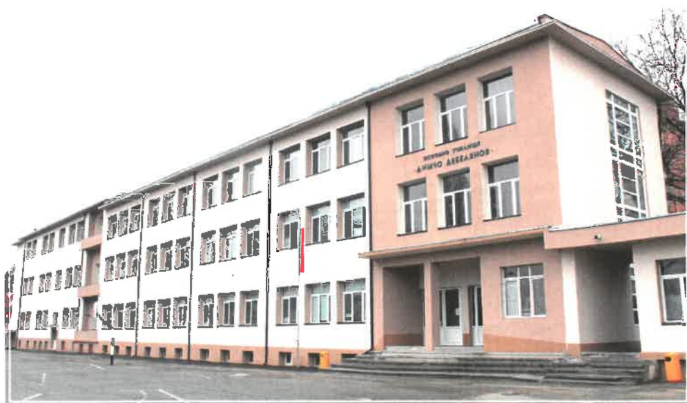
The renovated building of “Dimcho Debelyanov” high school in Yambol
