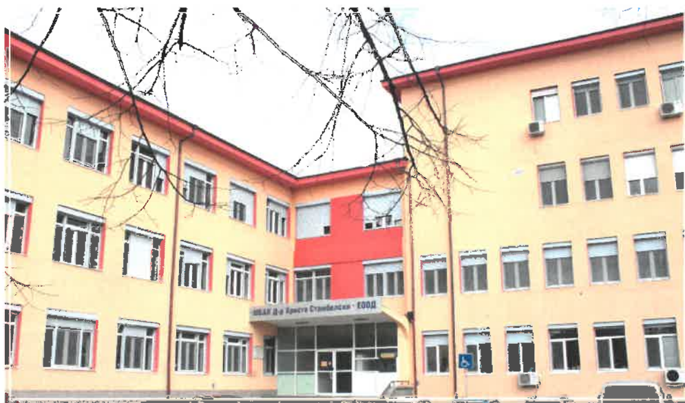
The renovated building of “Doctor Hristo Stambolski” multiprofile hospital for active treatment in Kazanlak.
